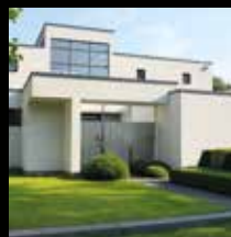
Find insulation problems
